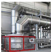
EcoReg® Rotary bed regenerator
